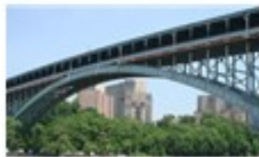
A metal bridge
